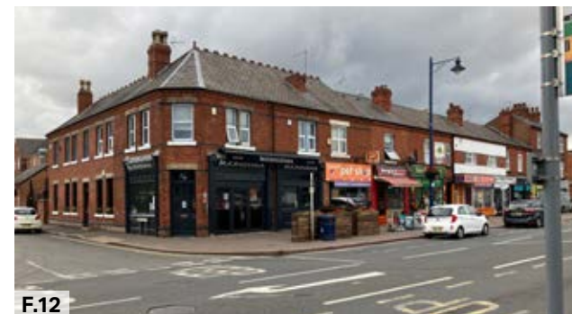
Figure 14: Mark Street provides existing site access
